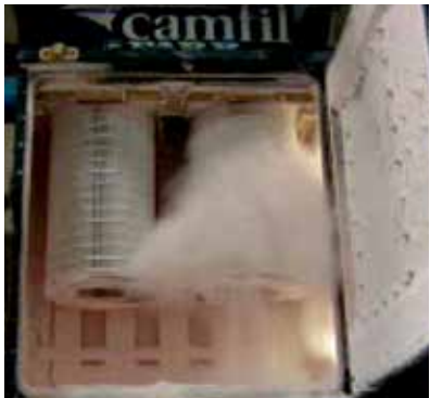
Pulse cleaning discharge of Gold Cone filter.
