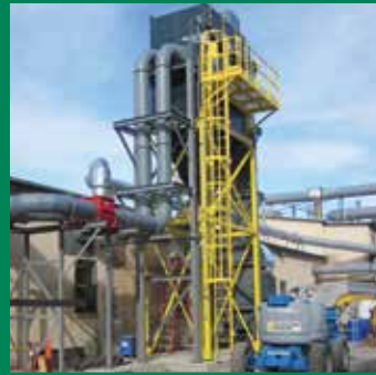
Heat Exchanger for Exhaust Gas that Cannot be Recirculated
